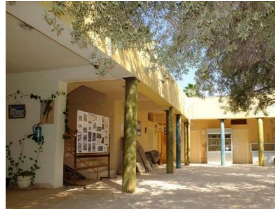
Deir Alla station in its new form
